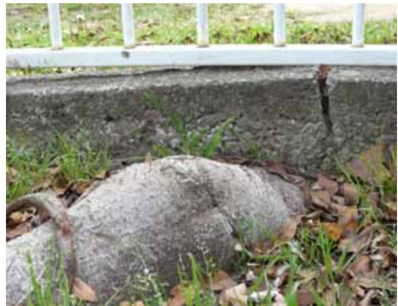
Above: Tree root damage to front fence, Block 2, Hastings Street
