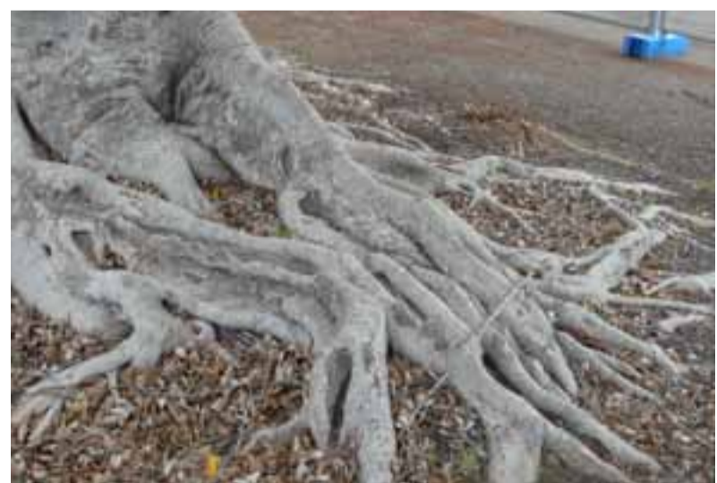
Above: Extensive unmanaged fig tree root growth in Block 2, Hastings Street
