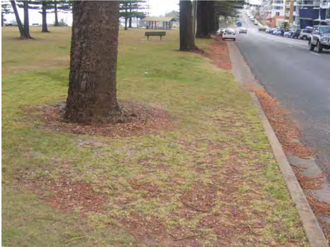
2. Adjacent Infrastructure corner Lord and William St. PMQ
